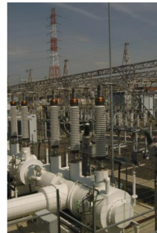
Fig. 2. TEPCO/Sumitomo 66 kV AC HTS test station at Asahi substation in Yokohama/Japan: left image shows the cable with a joint, right image shows the 66 kV AC end stations responsible for the transition from standard conductor to superconductor and from room to cryogenic temperature (2014).
